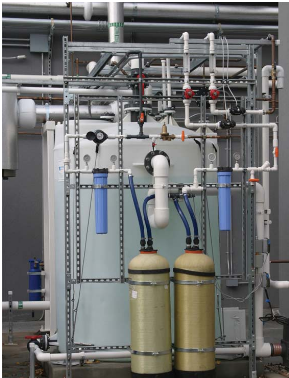
Dome Construction recently completed a cleantech LED Pilot Plant facility renovation in Newark.
